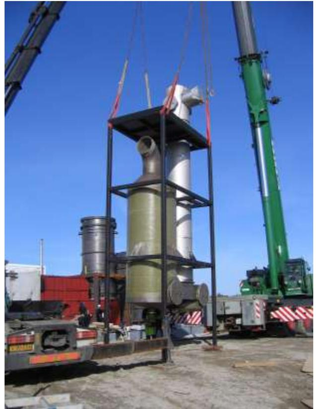
*The Condensing Unit (Scrubber) ensures that the final energy is pulled out of the flue gas.*
