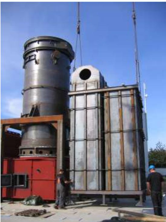
*20% of the power from the boiler and the enormous economizers, here inserted, turns into electricity.*
