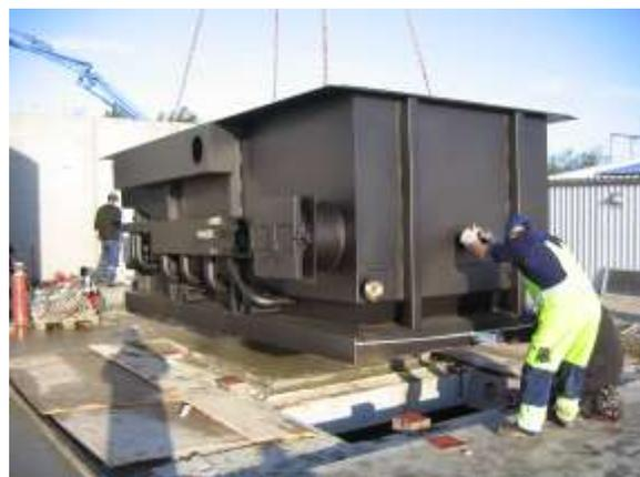
*Insertion of the water-cooled step grate, requiring great precision*
