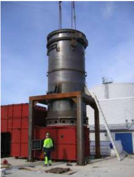
*Inserting of the oil boiler, which like the step grate is specially designed in collaboration with the Austrian Research Institute BIOS.*
